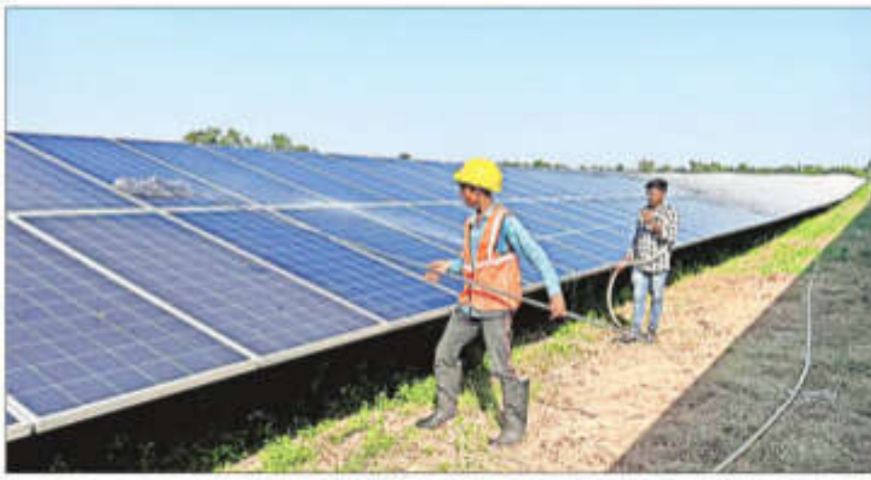
Agri-photovoltaics involves installing solar panels on elevated structures over agricultural land. REUTERS
