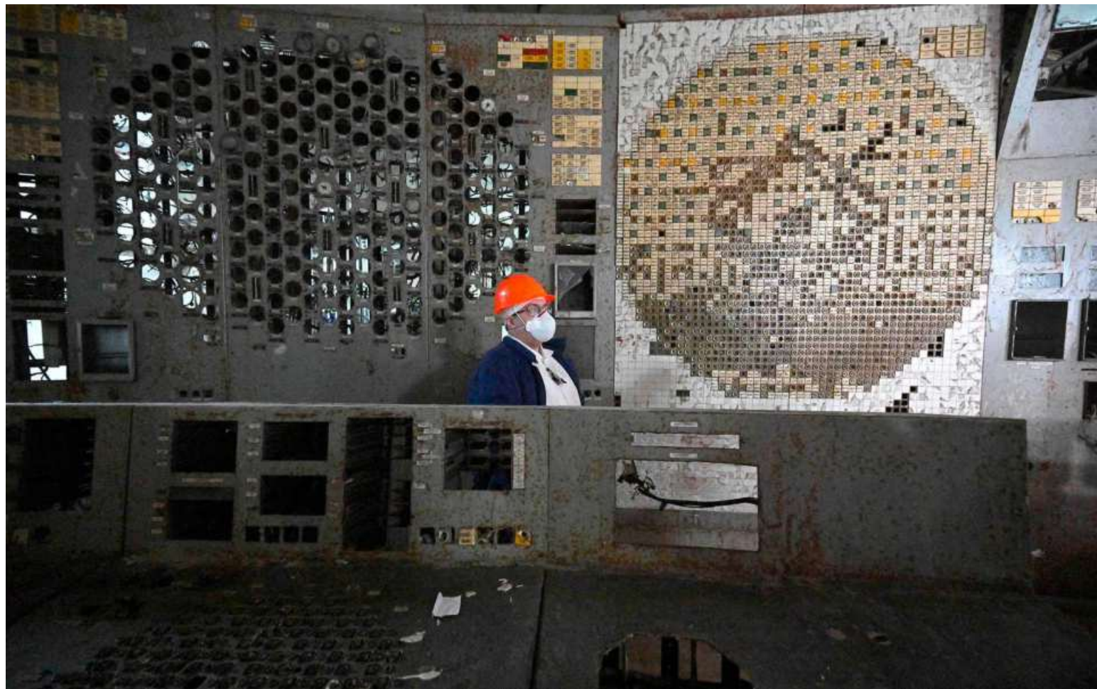
A view of the reactor core mimic display, a.k.a. the mnemonic table, that was part of the SKALA computer system at the Chernobyl nuclear power plant. By looking at the coloured tiles on the display, operators could quickly understand the distribution of activity across the core, helping them balance the reactor's power output and identify where heat was building up. AFP
